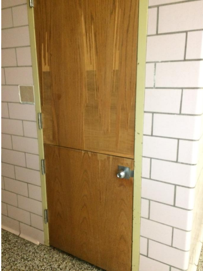
Interior Door in poor condition
