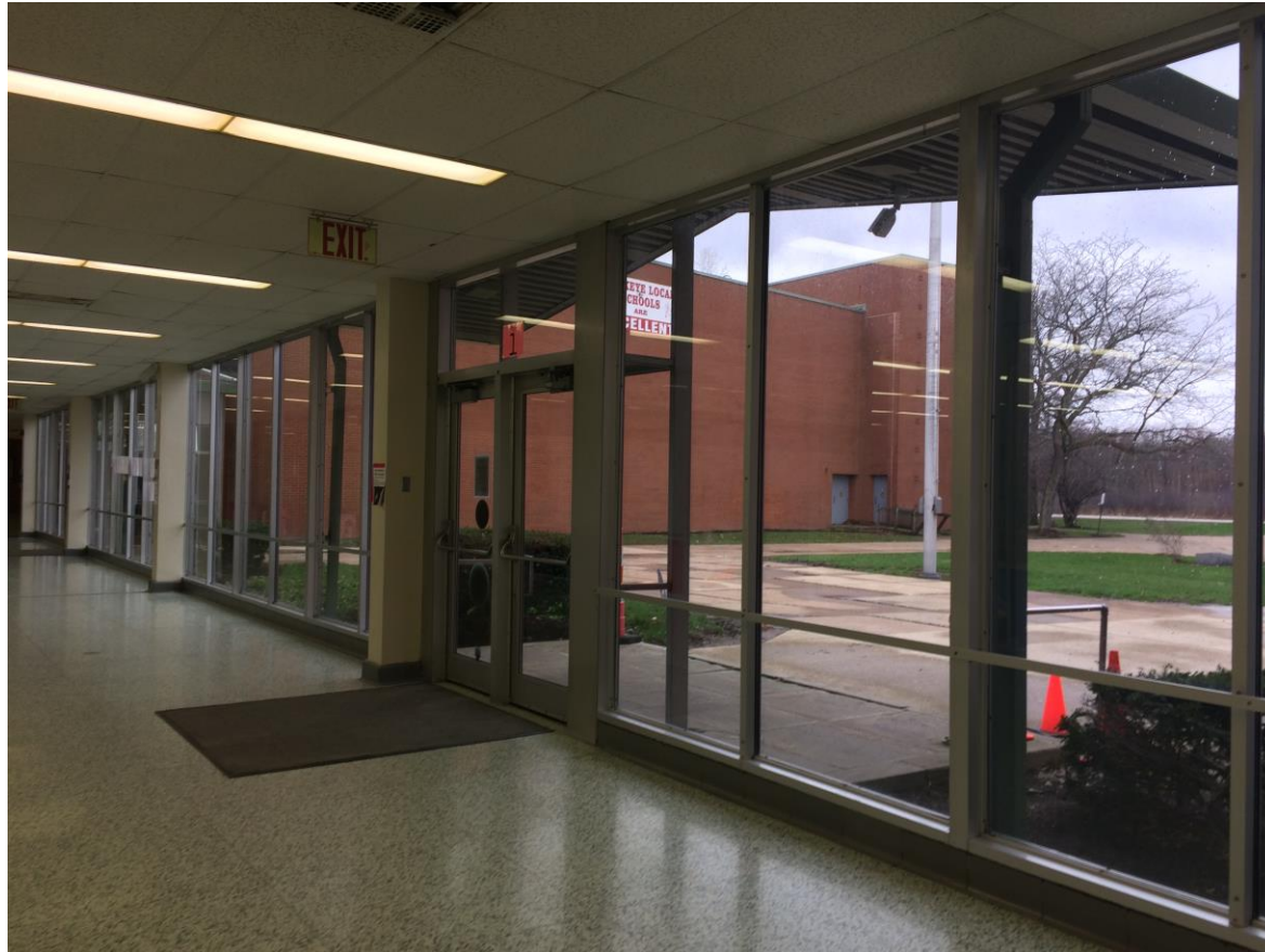
Main Entrance – Lack of Secure Vestibule
