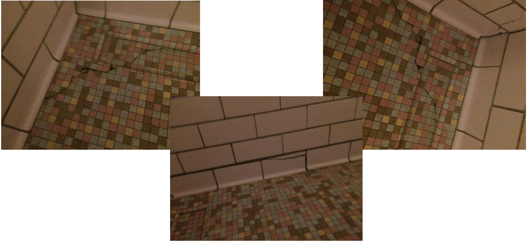
Floor sinking and wall cracking – shower rooms
